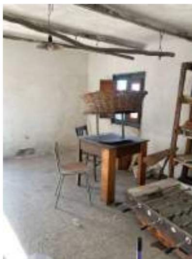
17: soffitta piano quarto
