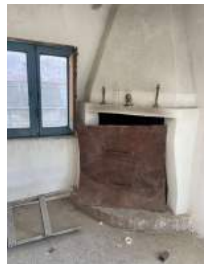
18: soffitta piano quarto
