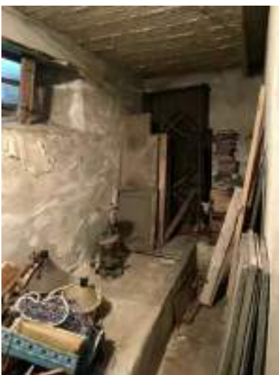
16: cantina piano interrato
