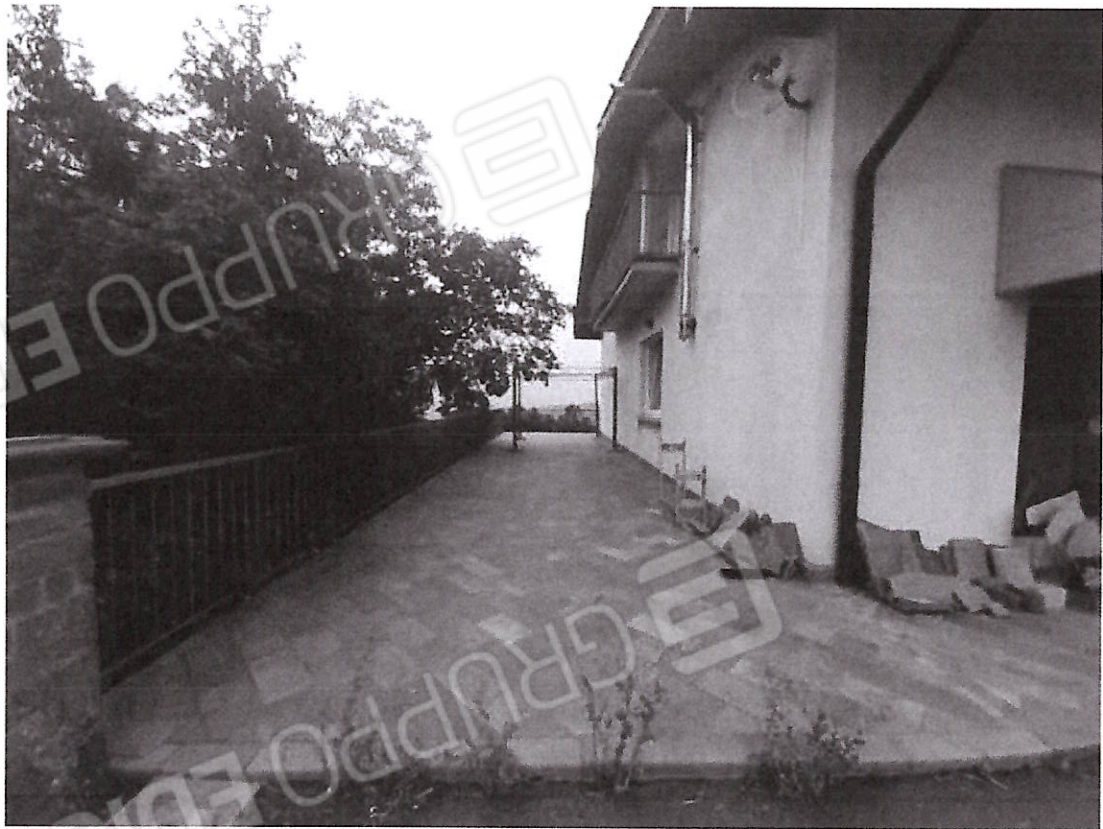
Vista rifiniture terrazzo e balcone in piano terra
